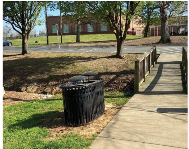
Address drainage issues throughout park
