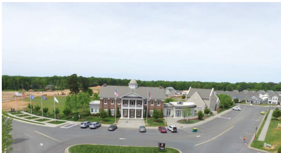
View over Locust City Hall under construction
