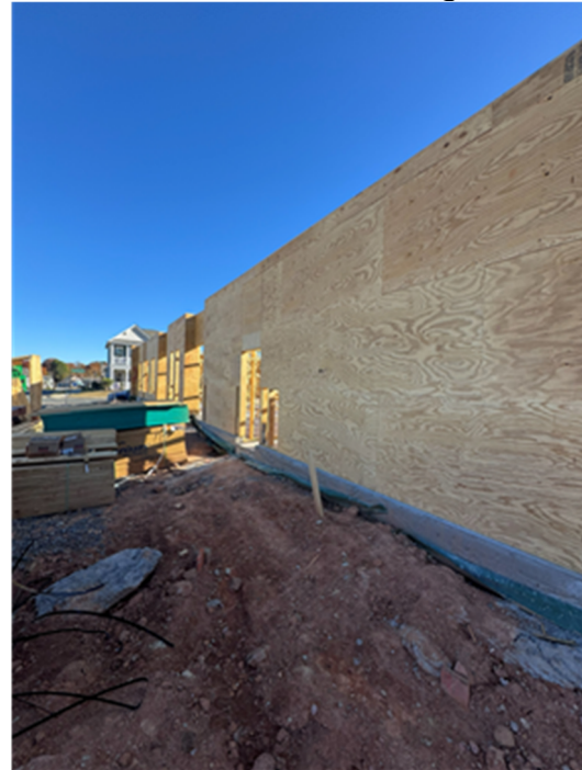
Exterior wall at rear of building
