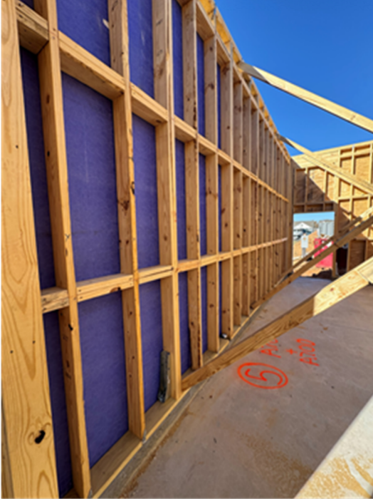
Men's Restroom Exterior Wall adjacent to existing Library. Type X sheathing installed at this location
