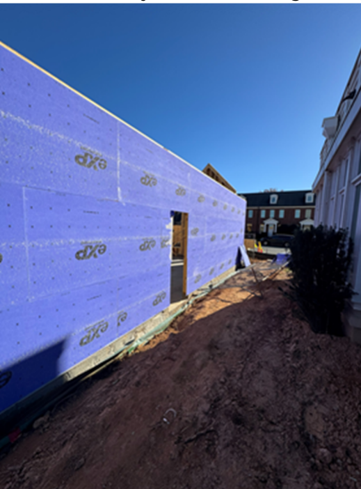
Exterior wall adjacent to existing Library.
