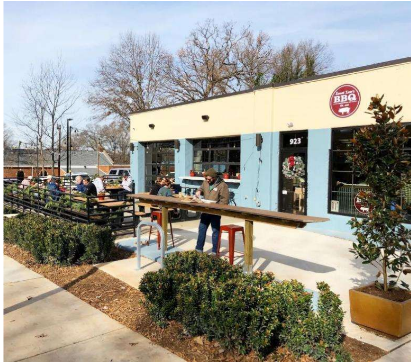
Before Tin Roof Covering
