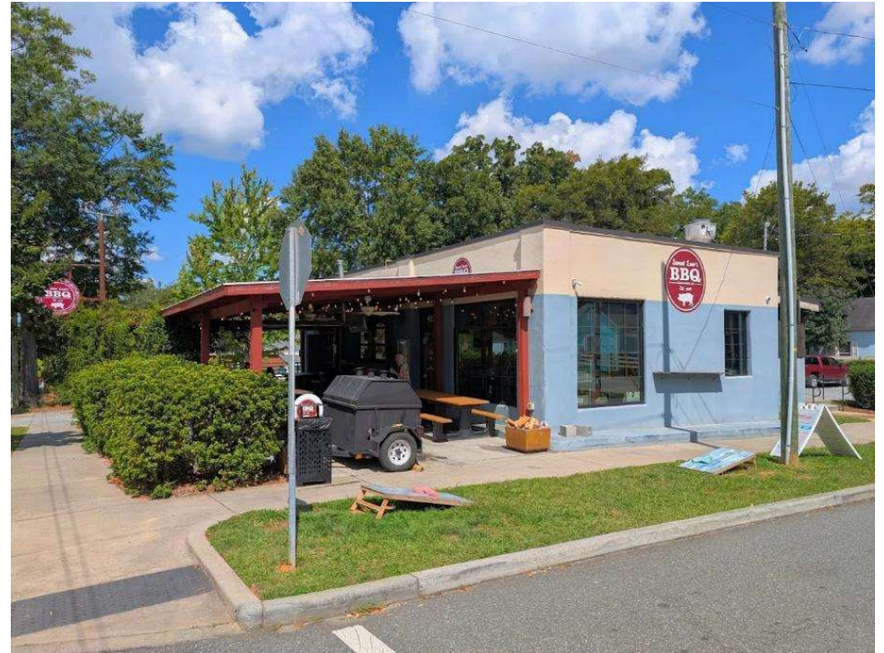
After Tin Roof Covering
