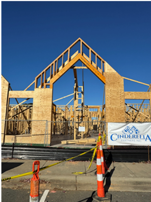
Main Entrance Gable end.
