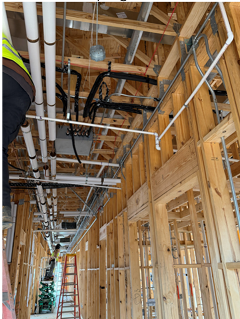
Corridor BS-1: Copper piping and insulation installation in progress.
