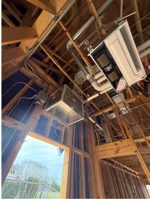
L2: Ductwork for Louver-2 installed.
