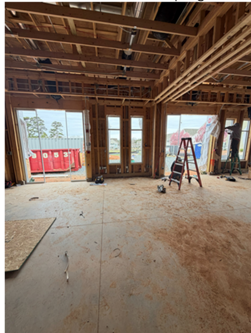
Installation of SF doors in progress
