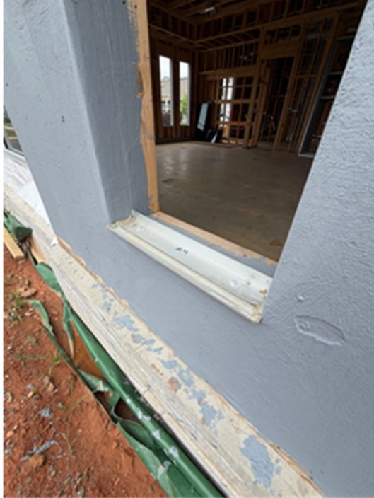
Reinstallation of Storefront Window frames.
