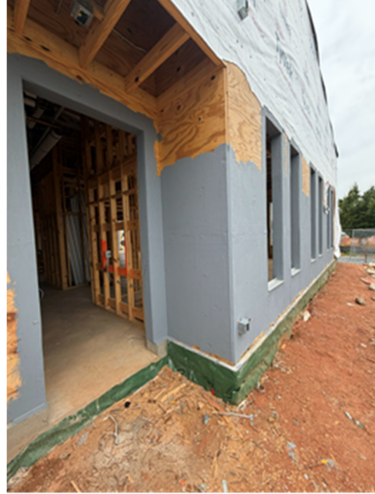
Liquid vapor barrier application on Kerri Dawn Lane.
