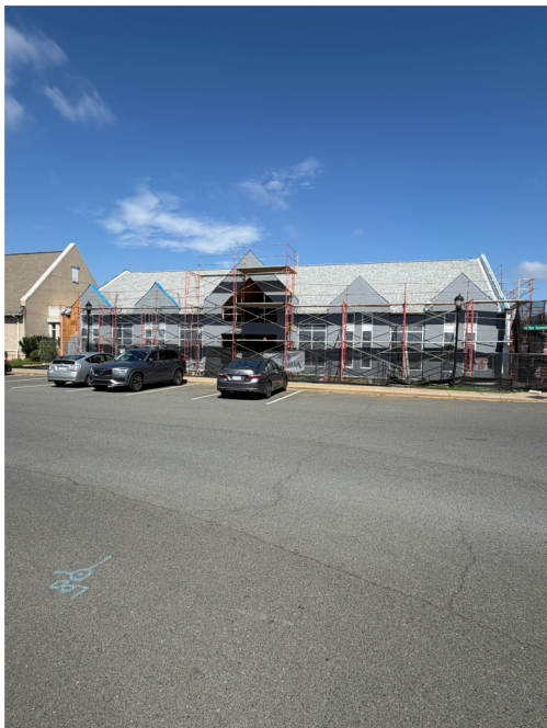
Liquid Barrier and foam boards installation in progress
