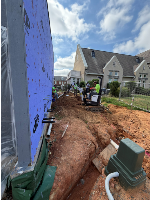
Piping installation for grease-trap in progress
