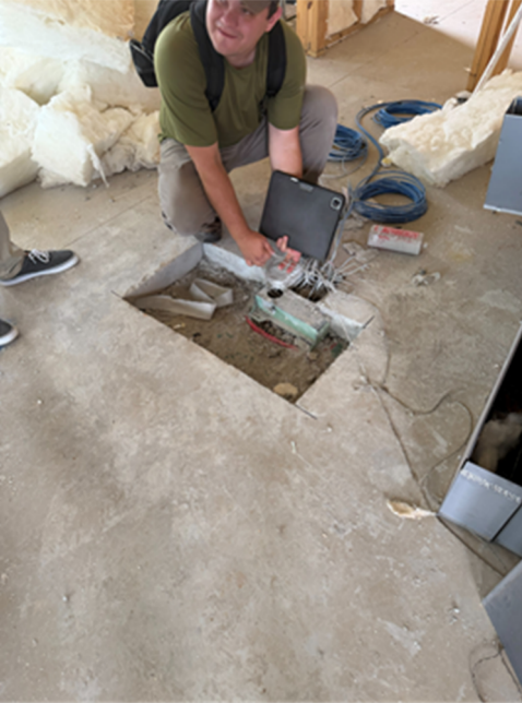
Work underway to remove rock in underground conduit.
