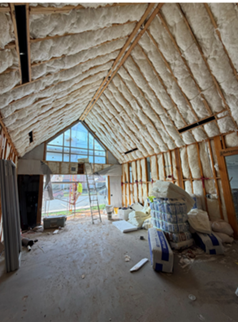
Lobby interior insulated. Entrance opening - delay in hardware for storefront doors. Openings need to be temporarily closed to protect interior (insulation) from inclement weather and to avoid delay in progress.
