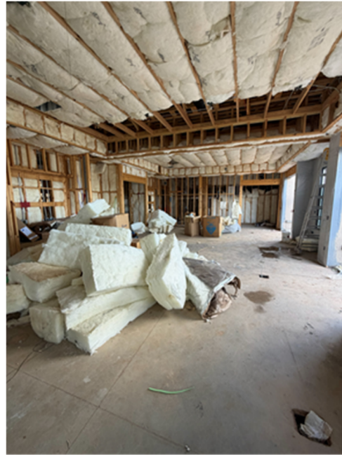
Interior insulation about 90% complete. Some had to be temporarily removed to run IT lines.
