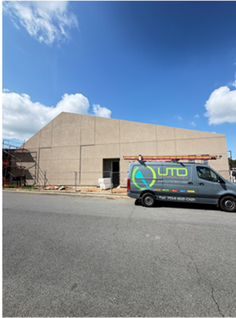
Exterior Elevation (Kerri Dawn Lane) completed.
