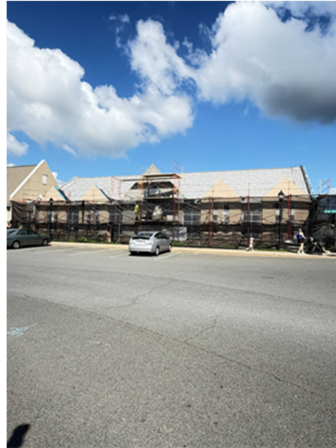
Exterior Elevation (Harrison Lane) - Finish lay in progress.
