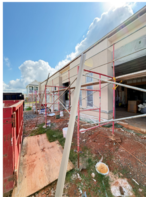
Multi-purpose exterior door openings. Openings are due to delay in hardware for storefront doors. Openings need to be temporarily closed to protect interior (insulation) from inclement weather and to avoid delay in progress. EIFS finish in progress.
