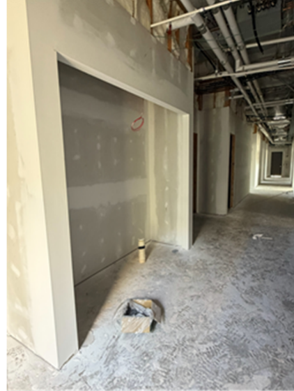
Drywall sanded and ready for painting.
