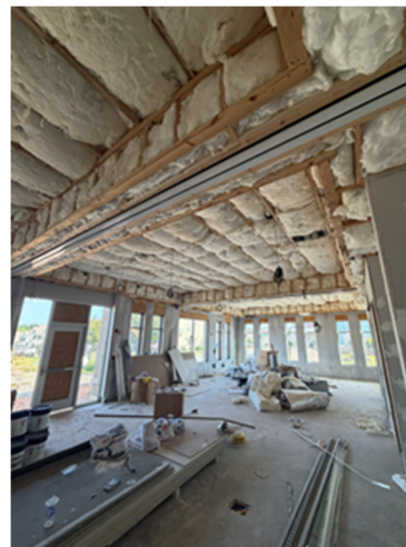
Multi-Purpose ceiling waiting inspection before Gyp installation can begin.
