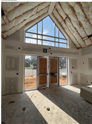
Main Storefront doors are installed.
