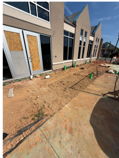
Grading at front of building. Underground storm drain piping installed.
