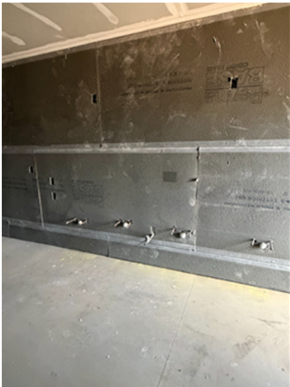
Restrooms ready to receive tile.
